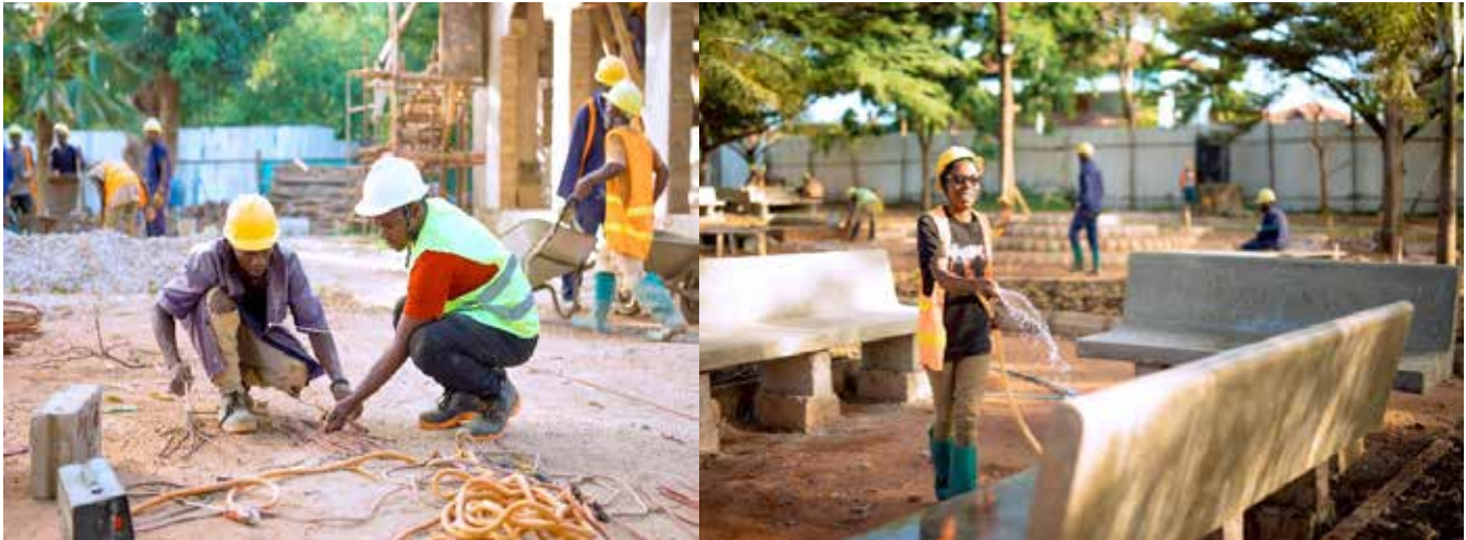
Technicians are at work in Redeveloping Jamhuri Park (Forodhani)
