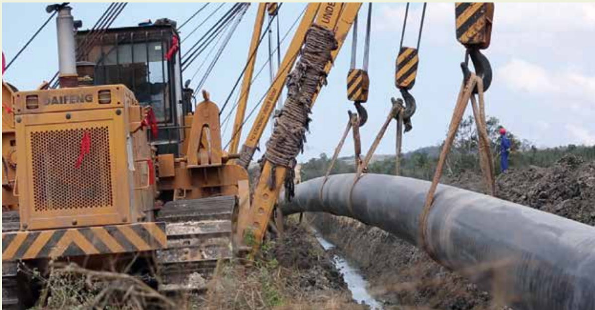
Construction of the gas pipeline from the Mandiba processing centre in Mtwara region to the commercial capital of Dar es Salaam.
